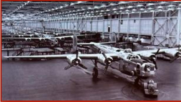
The first B-24 rolled off the line in June of 1942. One bomber was completed every 55 minutes. 8,865 bombers were built, over half of all B-24s constructed.
